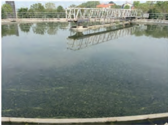
Ability improvement of the sewage disposal plant
